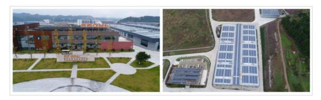
The PV power station is mounted on the production workshops, warehouse and office building of Nanchong Factory, amounting to an installed capacity of 1022.08KWp. The project adopts the model of self-use + grid-connect, where the surplus power will be sold to the national grid. Upon operation, the annual average power generation capacity of the station is up to approx. 1 million kW·h.
